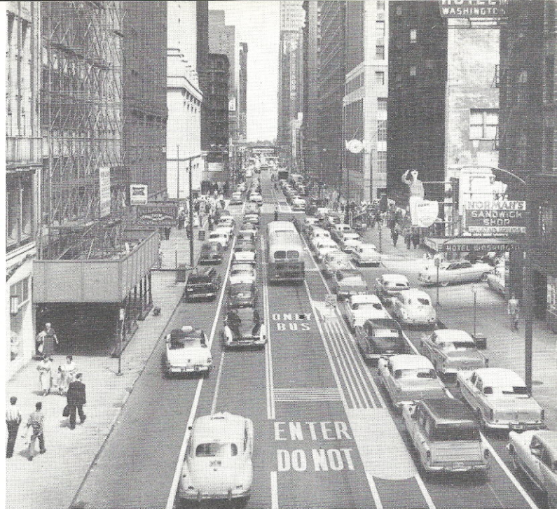
VIEW LOOKING EAST along Washington street from Wells street "L" Loop structure, showing clearly-marked exclusive bus transit lane in center of street. This picture demonstrates how an exclusive bus lane enables public transit vehicles to speed up schedules by eliminating mid-block traffic jams and delays even during non-rush hours.
