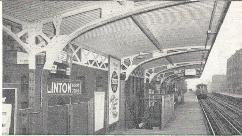
BRIGHTLY PAINTED walls, supports, railings, benches and overheads enhance the appearance of the Clinton street "L" station on the Lake street rapid transit line. Stairways and exteriors of this station, as on other stations of CTA's rapid transit system, are slated for similar treatment.
