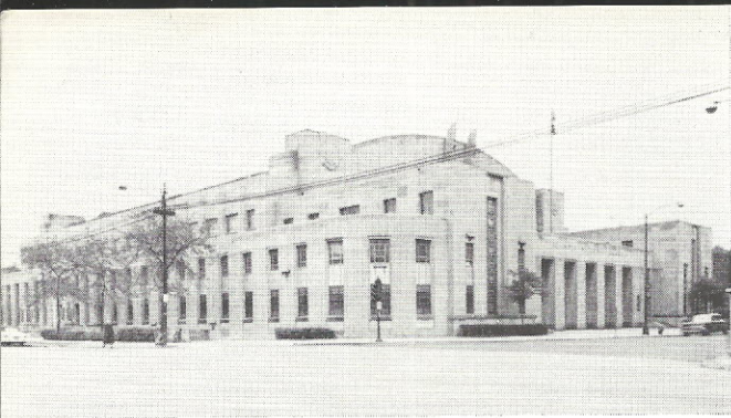
THE NORTHWEST Armory, at North and Kedzie avenues, is the headquarters of several Illinois National Guard units. The spacious structure, built in 1939, is a familiar sight to all riders on North avenue buses.
