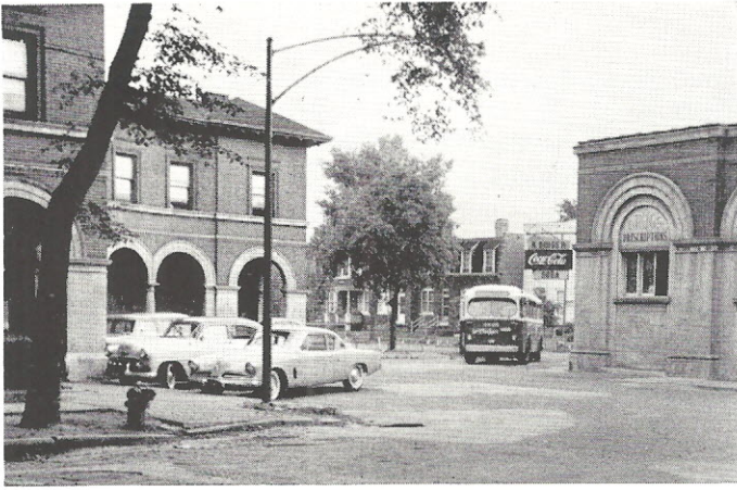
MANY OF the buildings of a "model town" complete with homes, store, church, school and theater, which were built in the 1880s by George M. Pullman for employes of his plant, still are in use today. Scene, within this "town," is at 112th and Champlain.
