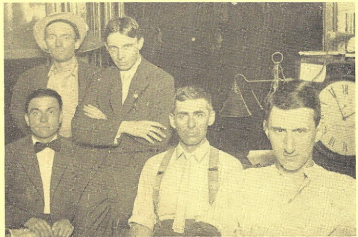
ONE DAY, back in 1914, these men took time out to have their picture taken at the Wilson avenue dispatcher's office of the old Northwestern Elevated Railroad. From left, in rear, are Motorman "Shorty" Farr and Towerman Carl Zimmerman. In front row, left to right, are Conductor Al Schiller and Towerman Ed Bartz. All are now deceased. Man at extreme right front is unidentified. The picture is the property of Towerman Henry Hengels, North Section.
