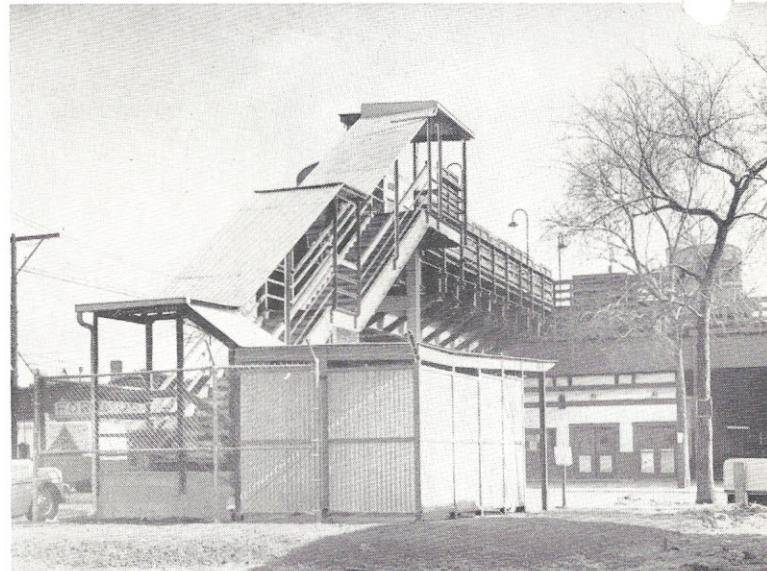
A NEW entrance-exit stairway at the west end of the 63rd-Loomis terminal station platform of the Englewood rapid transit branch was placed in service recently. An agent's booth is located in the small building in the fenced-off area at the foot of the stairway. This view looking east across Loomis street shows the main station in the background.
