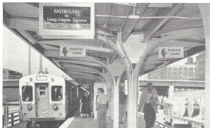
THIS VIEW shows the Halsted station platform on the new West Side Subway. Train is taking passengers on free inspection ride of new route on June 21. A two-aspect sign at upper left is controlled by switch in agent's booth. It indicates direction and destination of trains leaving from that side of the platform and when fares are paid on trains.
