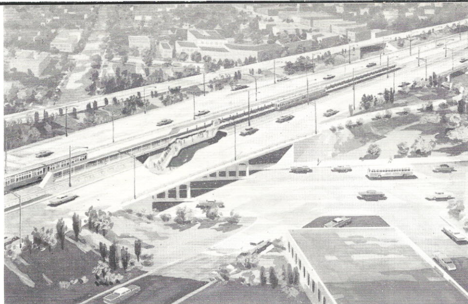
VIEW LOOKING west at the intersection of Pulaski and Northwest Expressway illustrates by cut-away the connections with the street at Pulaski road, the fare controls on the platform, and, in the background, the Irving Park boulevard entrances to the Pulaski-Irving station on the Northwest Expressway rapid transit.
