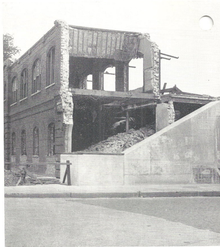
AS PART of the initial work on the Lake Street elevation project, the old North Western Railroad stations will be torn down. This picture shows the work in progress at the Austin avenue station, Parkside and Lake street, as it is being demolished. The retaining wall is being completed before total destruction of the building can take place.
