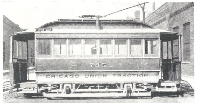
ONE OF the first electric cars to operate on the streets in 1893 was this bob-tailed trolley owned by the Chicago Union Traction Company. It is an old converted single truck car with a 15-horsepower motor and cost about $3,000. It could move at a maximum speed of 15 miles per hour. There were seats for 20 passengers who enjoyed the luxury of electric lighting and stove heat.
