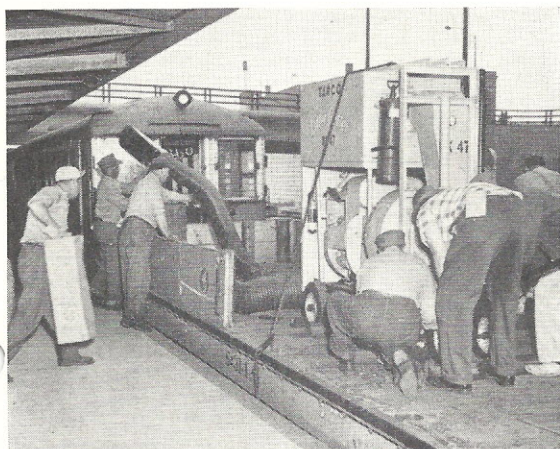
PARTIALLY DISASSEMBLED , the unit is moved from station to station on a flat car pulled by a work train. The suction hose has been detached and workmen are fastening down the steel case securely with ropes and wheel chocks.
