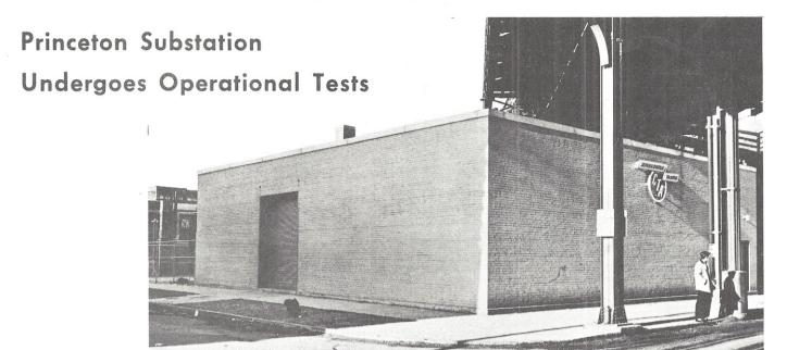
CTA CHALKED up another first recently when the modern Princeton substation went into test operation. To convert high voltage current into 600-volt traction power, silicon rectifiers are being used for the first time in rapid transit service in this country. Other transit companies now are showing great interest in the development.
