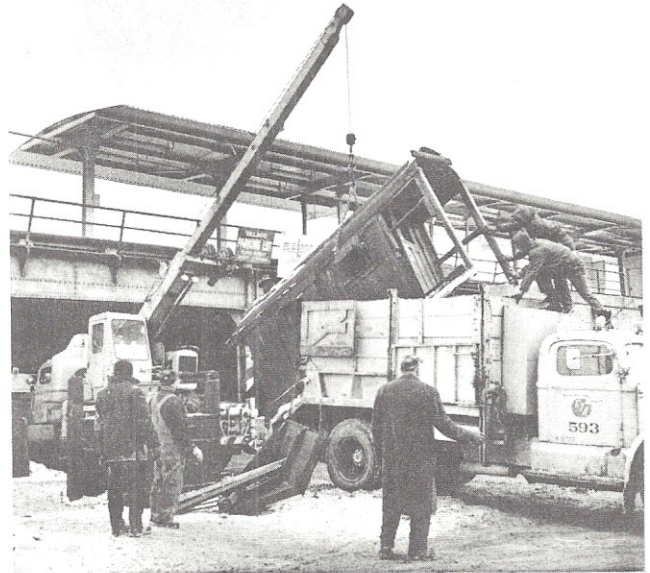
LIFTED FROM its foundation, the gateman's shanty at Oak Park avenue is loaded onto a truck for shipment to the Congress Terminal Shop, where it will be destroyed.
