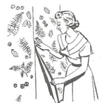
6. Put up next strip, "butting" edges and matching the pattern
