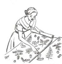
3. Match paper by placing one strip beside another
