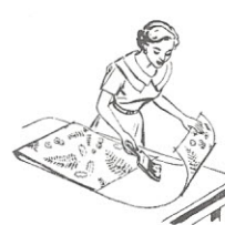
4. Apply paste evenly, fold pasted end toward center, paste other end
