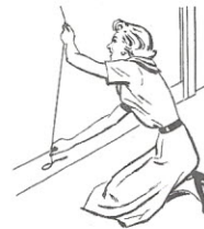
2. Use a plumb line to get first strip of paper straight
