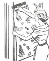
5. Hang first strip on wall, smooth down with handy brush
