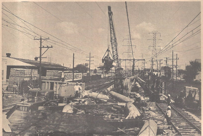
TO PROVIDE greater visibility at street crossings, unused stations and island-type platforms have been removed from the grade-level portions of the Skokie Swift route. The stations not only impaired motormen's view of the crossings, but also were unsightly and an attraction for children. Demolition of the old Oakton street station (below) was completed Sunday, May 10; the unused Kostner station (left) was removed the following Sunday.
