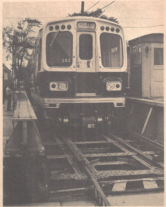
TO PROVIDE greater visibility at street crossings, unused stations and island-type platforms have been removed from the grade-level portions of the Skokie Swift route. The stations not only impaired motormen's view of the crossings, but also were unsightly and an attraction for children. Demolition of the old Oakton street station (below) was completed Sunday, May 10; the unused Kostner station (left) was removed the following Sunday.
