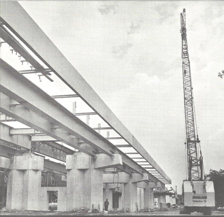
A **BREAKTHROUGH** in the design of elevated structures was achieved on the Englewood rapid transit project through the combined use of concrete and steel. Photos here show contractor completing work in various stages along the extension west from the present Loomis terminal to the end of track near Hermitage avenue:
