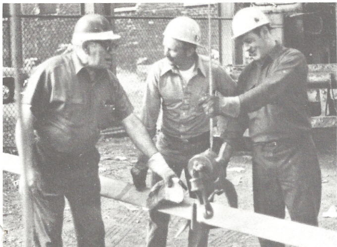
Reader instructs Ironworkers Bernard Keller (center) and Sean Brady in the hookup of a flange angle before it is raised to the scaffold.
