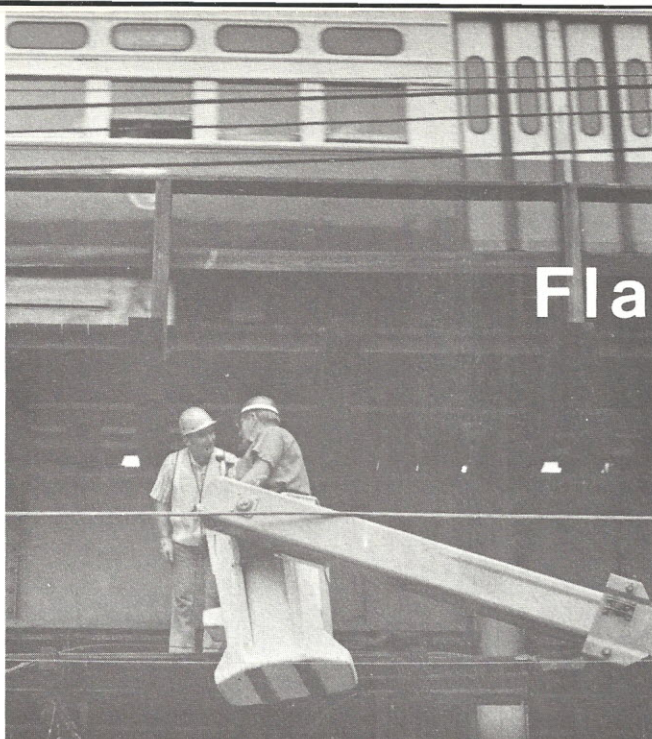
Trains going by overhead are just "part of the job" to Kilroy and Reader as they check to see which angles need to be replaced.
