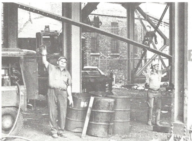
Reader and Keller guide the hoisting of a flange angle to the scaffold.
