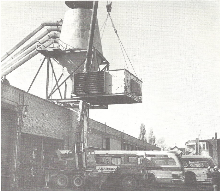
HEAT TO THE ROOF: Swinging to the roof of the Archer garage is the first of two new heaters with a 2.5 million BTU capacity per unit. The new units replace two smaller heaters which had been used for 10 years. Steel structure of the building was altered to accommodate the larger units and new wiring was installed. The $45,000 project also includes improved heating in the bus fueling and washing bays.
