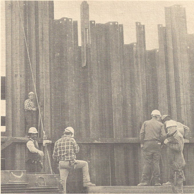
AT DESPLAINES: The new terminal construction project is underway. The temporary parking lot for commuters has been opened. Steel sheet piling is being installed to hold back the earth which will support the temporary station and tracks. This permits excavation to a depth of 15 feet for the foundation for the new terminal.
