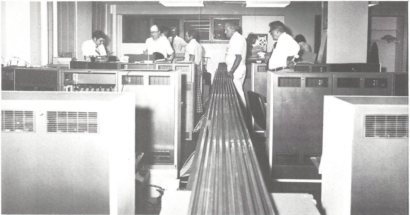
Inspecting new equipment for bus controllers are (from left) John Farar, program manager of Motorola Communications & Electronics, Inc.; George Krambles, CTA general manager; Robert Davis, a vice president of Motorola, and Al Sterland, a national sales manager of Motorola. The long piece of equipment is a message conveyor.
