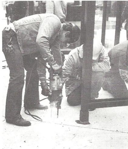
Drilling holes into concrete for bolting shelter to sidewalk.
