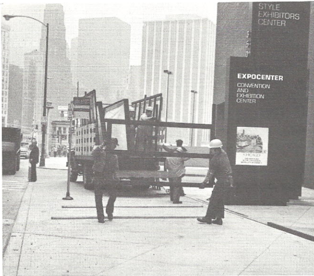
Unloading the prefabricated section of the bus passenger shelter.
