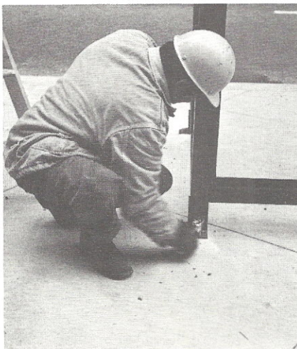
Bolting the shelter to the sidewalk.
