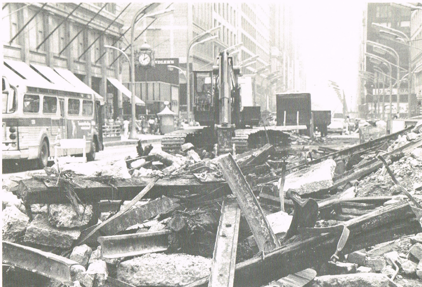
Old streetcar track is turned up as excavation begins for State Street Mall.
