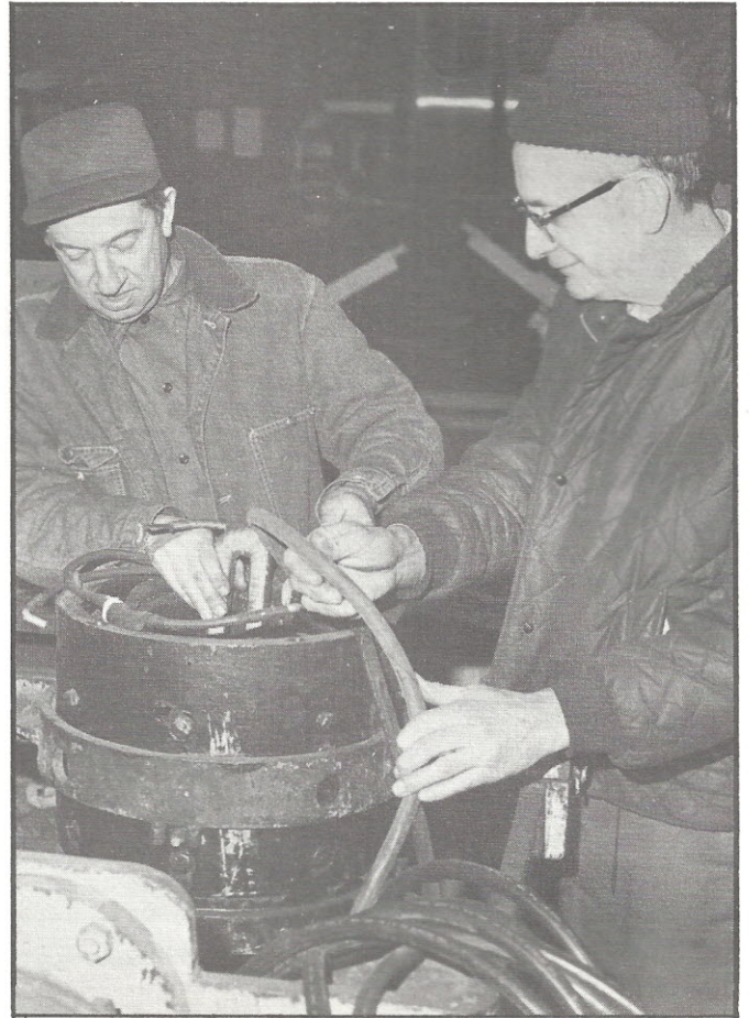
Lino Lupetini and Casimer Turek install field coil.
