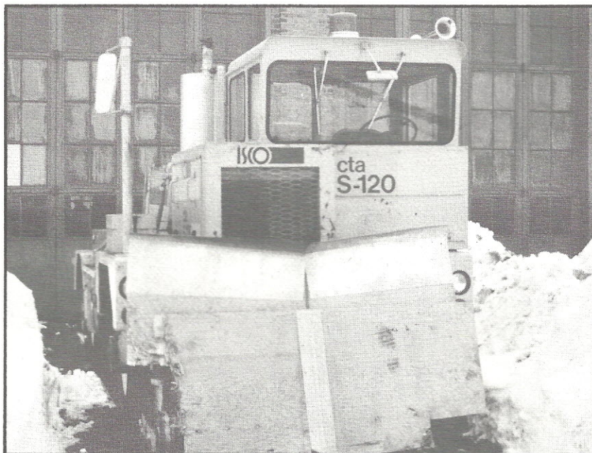
Diesel powered plow, operable on rail or pavement, was used to clear Skokie Shop area and part of Skokie Swift route.
