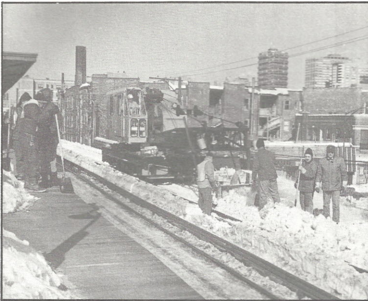
Blower mounted on crane to remove snow between rails at Bryn Mawr station, Feb. 7.
