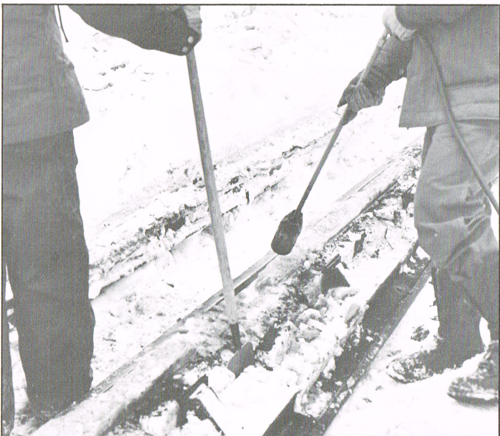
Melting ice with propane torch on Evanston branch, Jan. 19.
