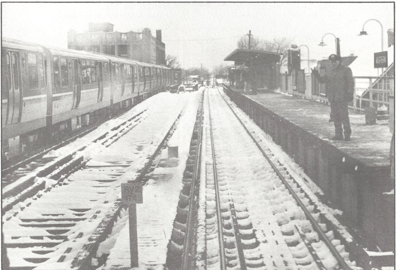
Western station on Ravenswood, Jan. 15, an example of how excessive snow did not accumulate on elevated structure.
