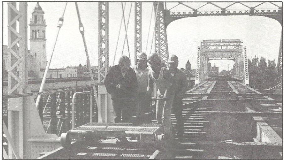
Removing rapid transit tracks from the bridges.
