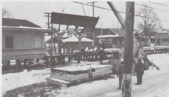
Crane is used to remove portions of the station canopy.
