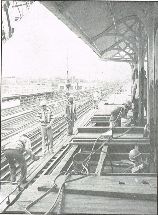
Rehabilitation work at King Drive shows track crews preparing for rail installation while ironworkers repair steel platform canopy supports.
