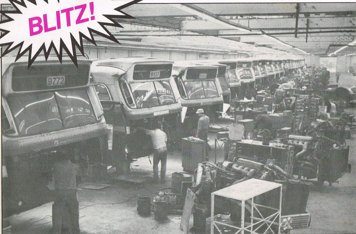
Row of CTA buses in Blitz's remanufacturing shop on the West Side. Old, damaged bulkheads and rear assemblies are being removed following dismantling of engines and transmissions.
