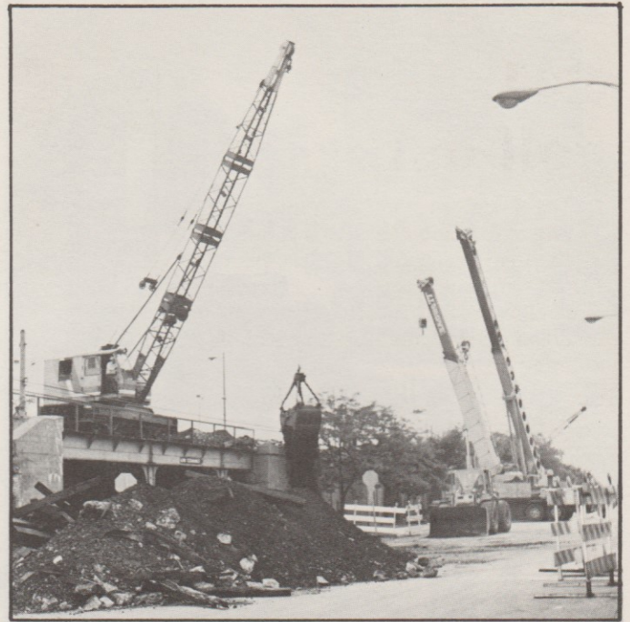
CTA crane removes 600 tons of ballast from Lake elevated embankment onto Lake Street at Marion Street, Oak Park.
