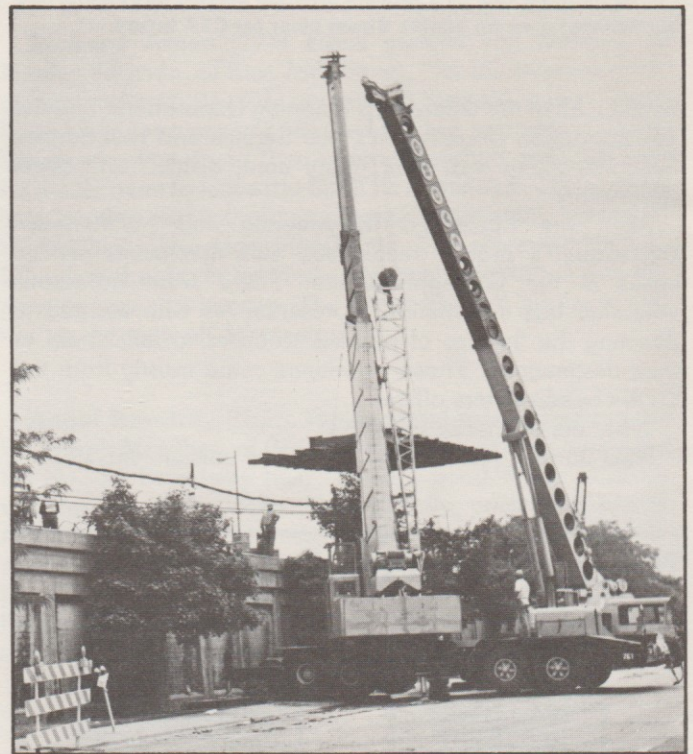
Contractor's cranes hoist 34-ton diamond crossover component from truck onto 'L' embankment.
