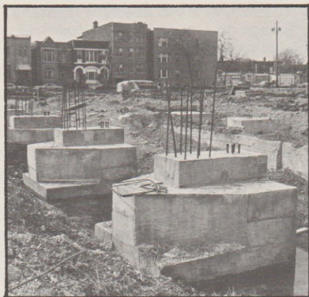
The new Kedzie garage construction project has progressed from pile caps (left) to steel frame, and is scheduled for completion in March, 1984.
