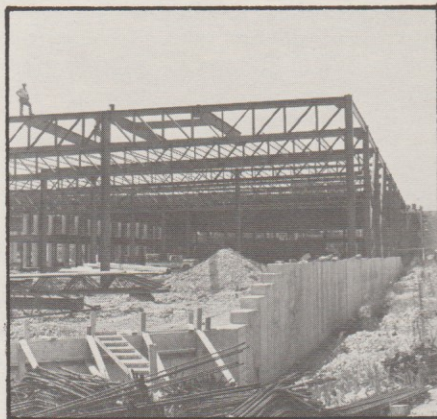
The new Kedzie garage construction project has progressed from pile caps (left) to steel frame, and is scheduled for completion in March, 1984.
