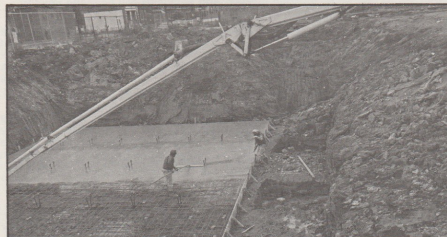
This excavated site with its sub-grade work will be the tank pad with a capacity to store 100,000 gallons of diesel fuel.
