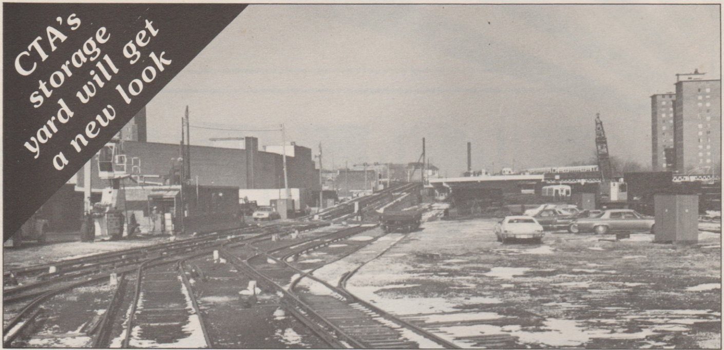
View of present Lower Yard with electric powered third rail-system. Concrete incline is in center of photo.
