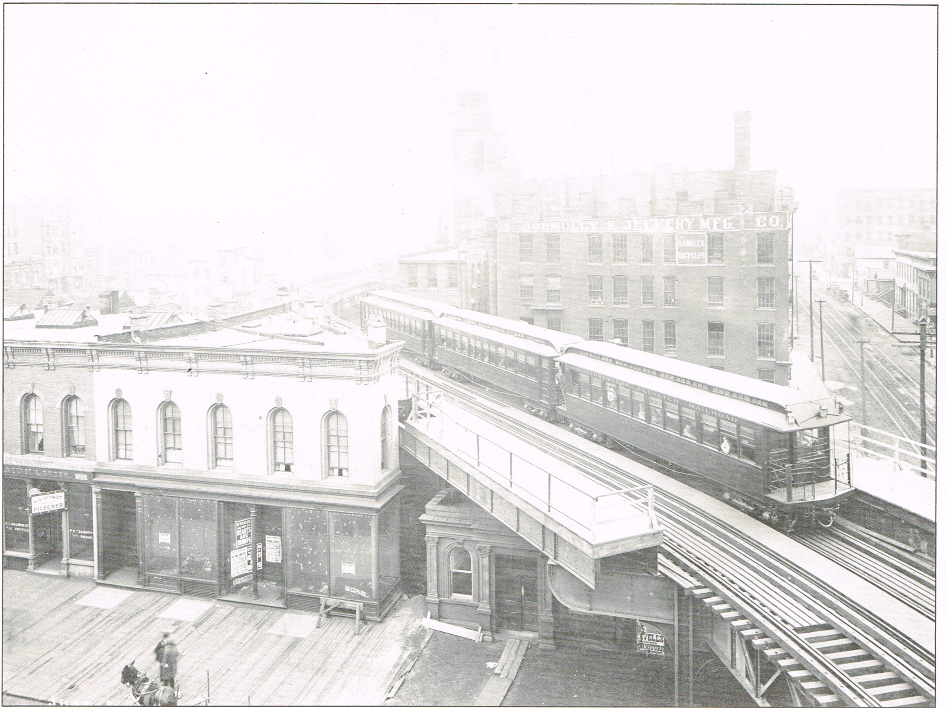
Pullman-built cars of the Northwestern Elevated Railroad, like this train at Chicago Avenue, ran on the left side when service was started in 1900.
