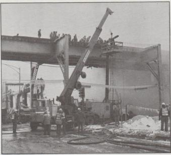
A Bantam crane and tower truck hoists men and material up to build new track at Lake street. Extensive repairs were needed following firemen and CTA workers' around-the-clock efforts to subdue a multialarm fire which temporarily halted "L" service.
