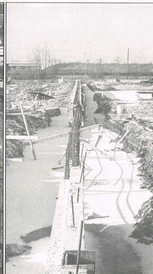
South wall shows more progress on grade beams after concrete has been poured.
