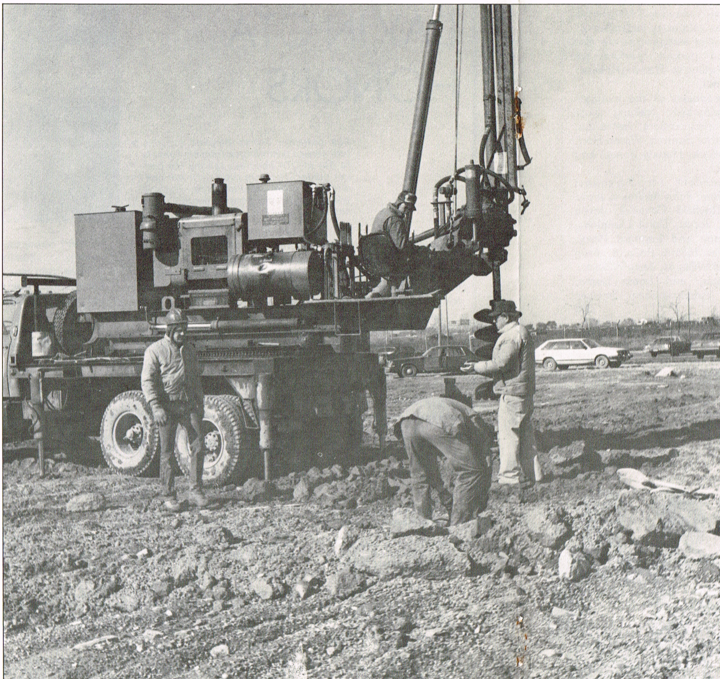
Specialized equipment is used when drilling for one of the 246 caissons that will form the subgrade foundation for the garage structure.
