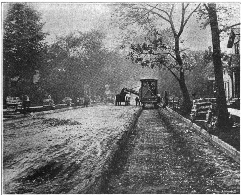
"The Passing of the Pick and Shovel." Koehring Rotary Grader at Work
