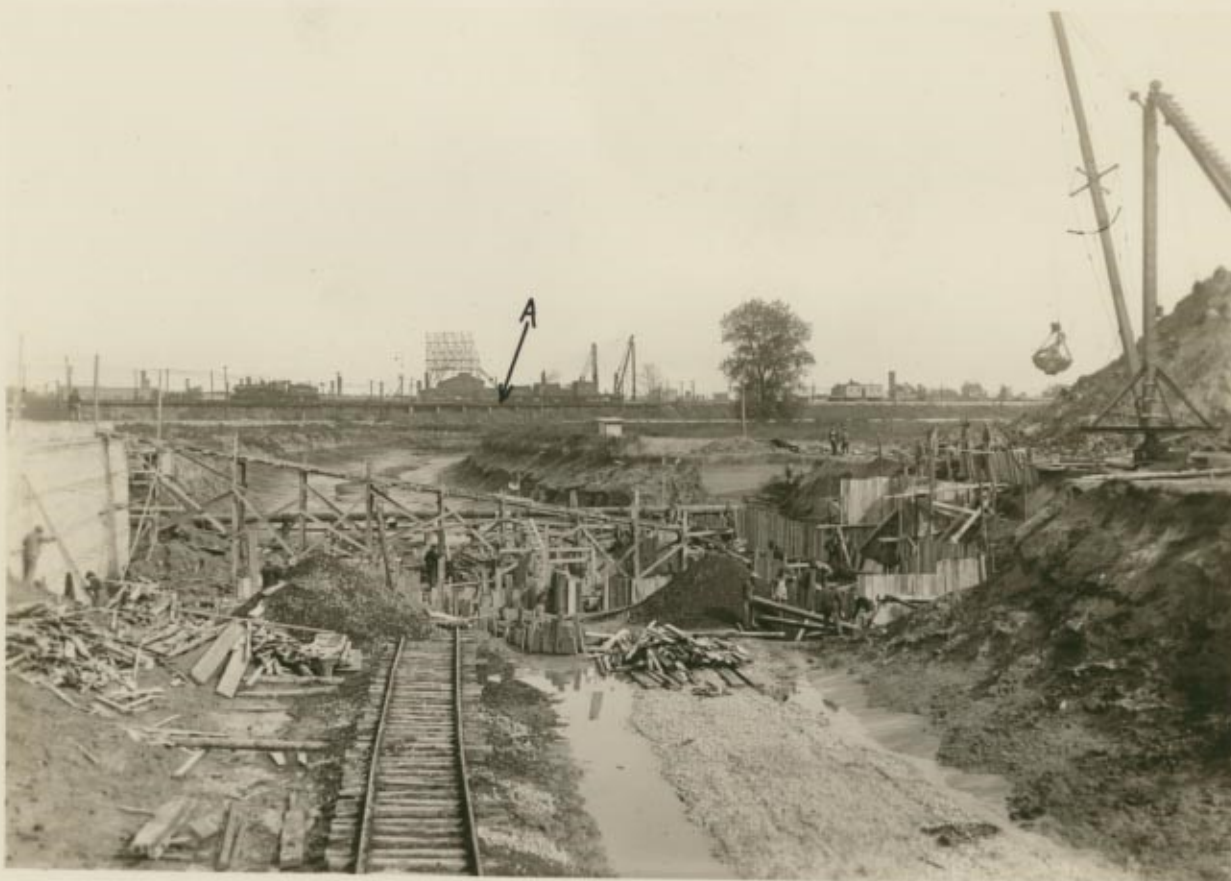
Looking east September 30, 1924 from the future Custer Street bridge, on the Skokie Valley Line, and showing a section of the roadbed, which at this place averages about 12 feet in depth. At the point marked "A" the new line will pass between the main line of the Milwaukee division of the Chicago and Northwestern railway, and a crew may be seen driving piles preparatory to beginning construction of the subway. In the foreground are construction facilities for the Custer Street bridge over the new line.
