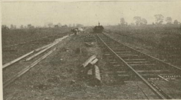
Laying permanent track on Niles Center Extension
