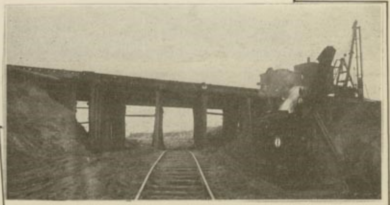
Laying permanent track on Niles Center Extension
