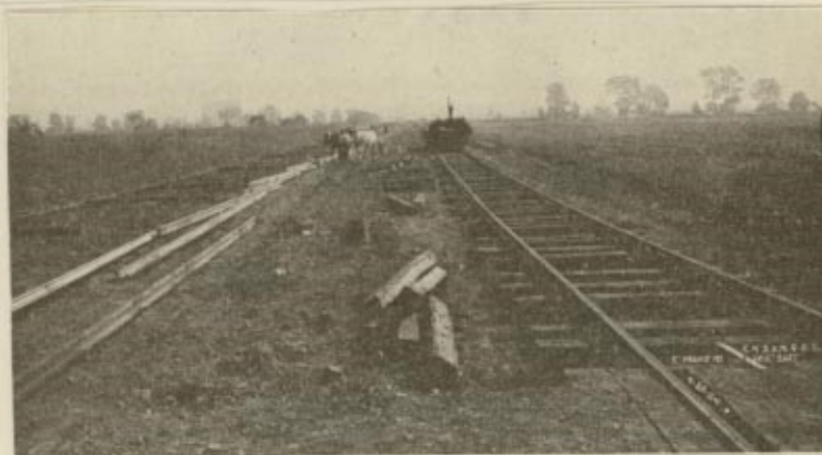
Laying permanent track on Niles Center Extension
