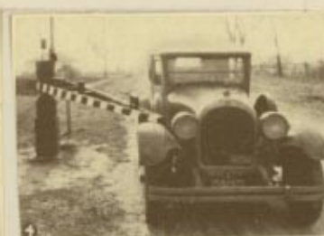
(4) Gate being swung aside by automobile failing to stop
