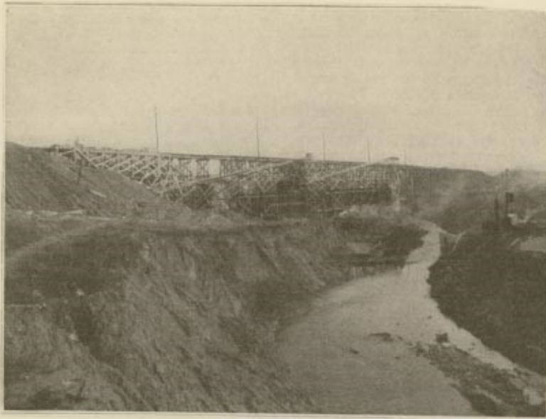
Starting excavation for culvert at Kinnickinnick River over Madison Division of the Chicago and Northwestern Railway tracks.
