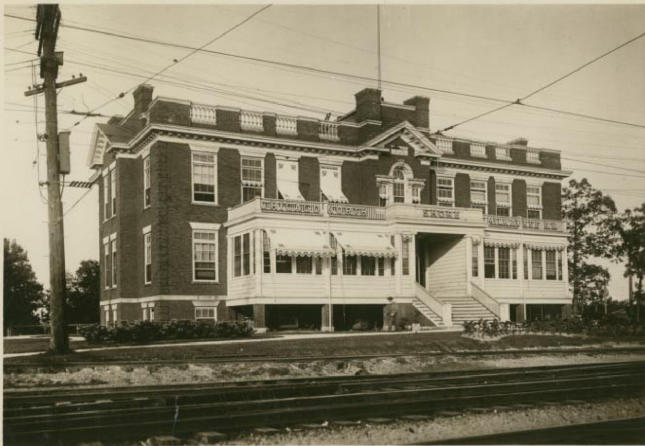
Front or West view of the general offices of the North Shore Line at Highwood, Illinois. The two-story and basement brick building is 40 feet by 90 feet, and is still occupied by general offices and lunch room. This building was erected in 1905 and in its immediate vicinity are carbarns, yards and recreation rooms for employes.
