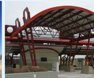
Northwest Transportation Center
