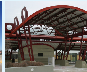
Northwest Transportation Center
