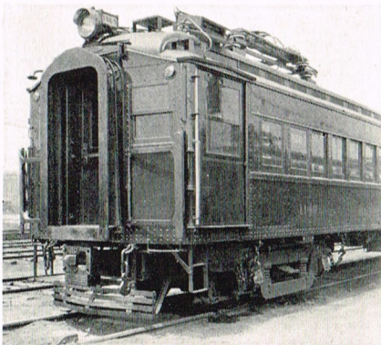
Illinois Central light-weight suburban cars built in 1923.
