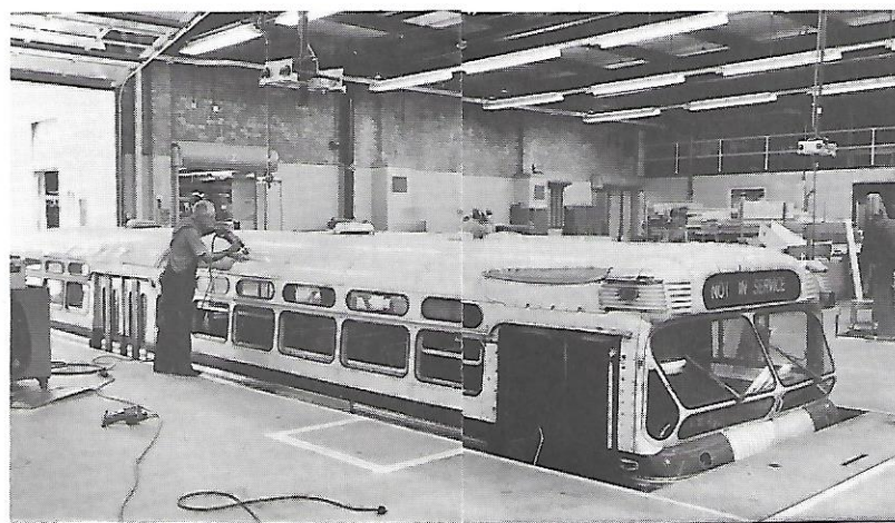
Twenty-eight hydraulic hoists elevate buses for replacement of major underbody components in the chassis shops.
