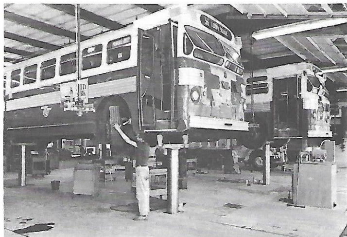
Twenty-eight hydraulic hoists elevate buses for replacement of major underbody components in the chassis shops.
