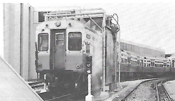
The automatic car washer at the Congress Terminal shop can wash an entire train sparkling clean in minutes.
