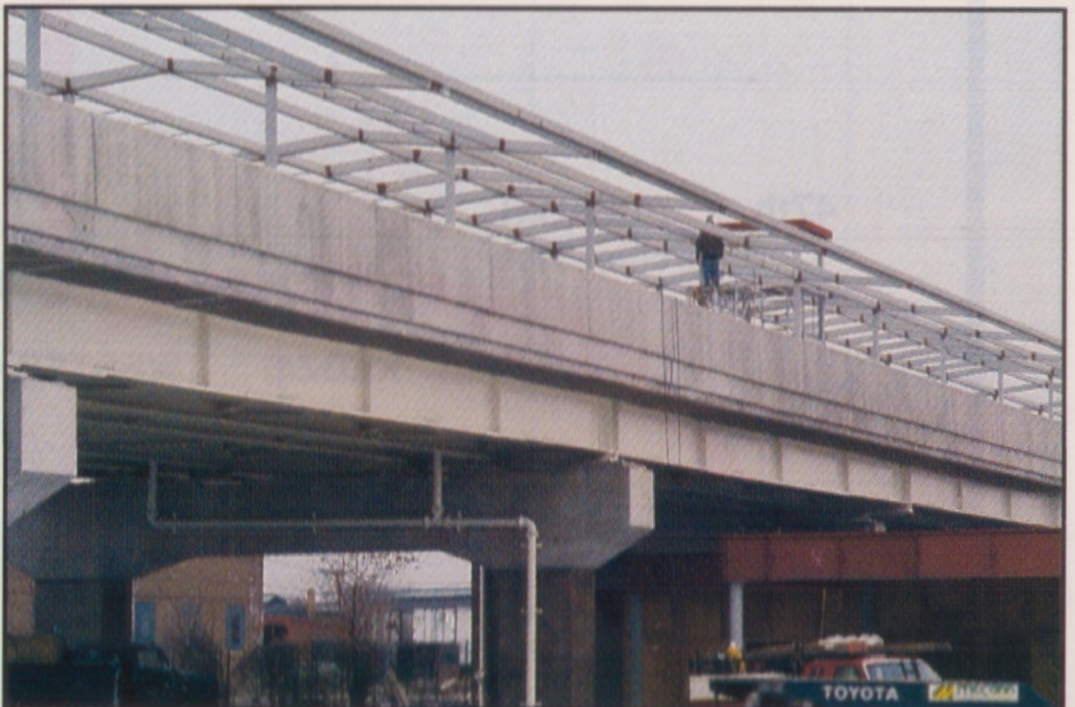
Canopy under construction at Pulaski/Archer Station
