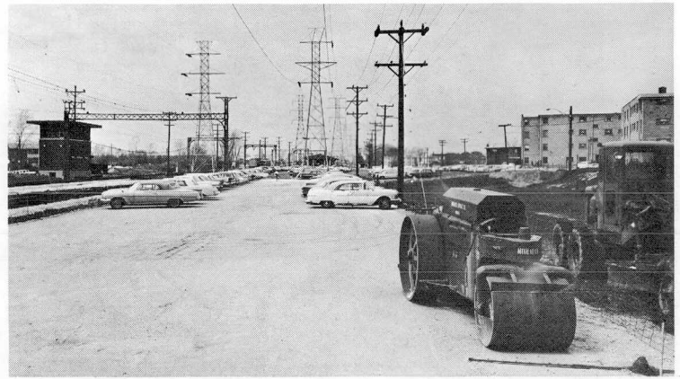
64-car addition to park-'n'-ride lot being rushed to completion late in April to handle overflow immediately experienced upon opening of project. Binder and finish courses will be applied in second quarter.
