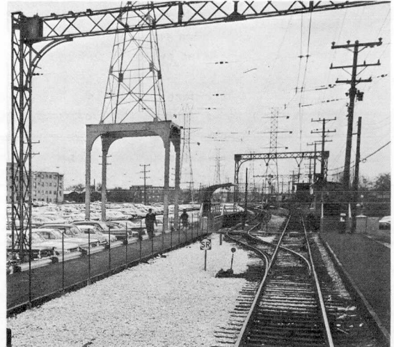
New Switch and trolley wires installed at Dempster Station.
