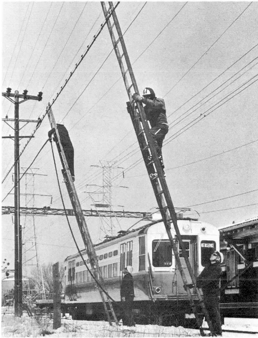
Linemen installing new cable at Dempster Terminal. Test train in background checking trolley wire alignment.
