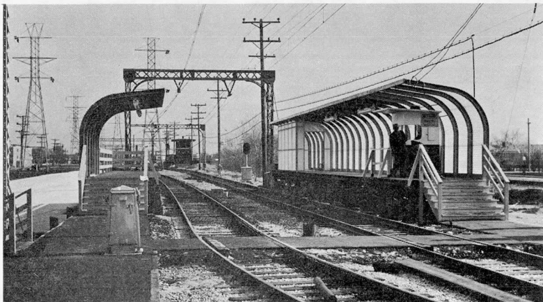
Two views of new Dempster station platforms under construction. Short platform accommodates arriving trains, while larger platform with booth serves southbound traffic.
