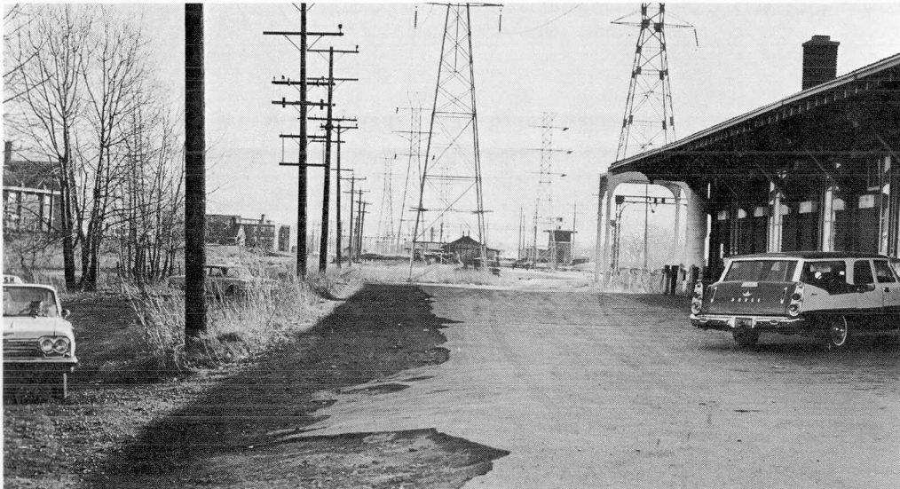
The very small part of the park-'n'-ride area which had been paved by the predecessor railroad, poorly graded and in bad condition, had to be torn out along with old frame buildings seen in the distant background. Photo below shows grading in progress.
