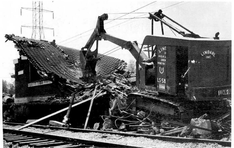
Demolition of four unused stations and high-level platforms, which impaired motormen's view at grade crossings, was accomplished on Sundays during May and June. Pictured here are two stations in the process of being razed on Sunday, May 10; at the left, the wrecker's ball is being used to break up the concrete platform between Crawford avenue and East Prairie road; above, a dragline is working on the station building at Kostner avenue.
