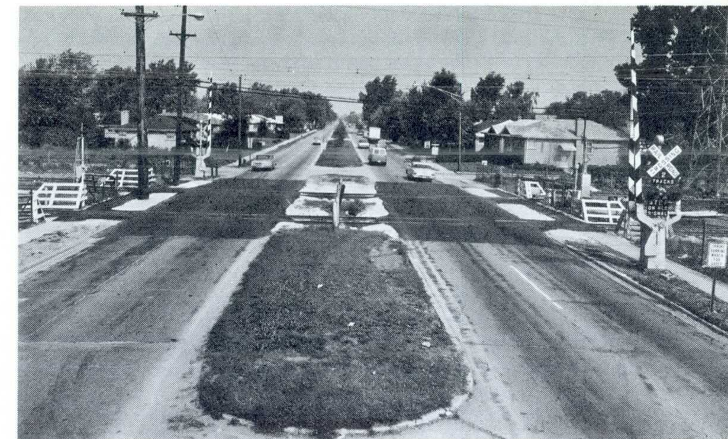
Tracks and pavement at Crawford crossing were completely rebuilt during the quarter to correct deteriorated conditions that had been reflected in excessive roughness for both trains and motor vehicles.
