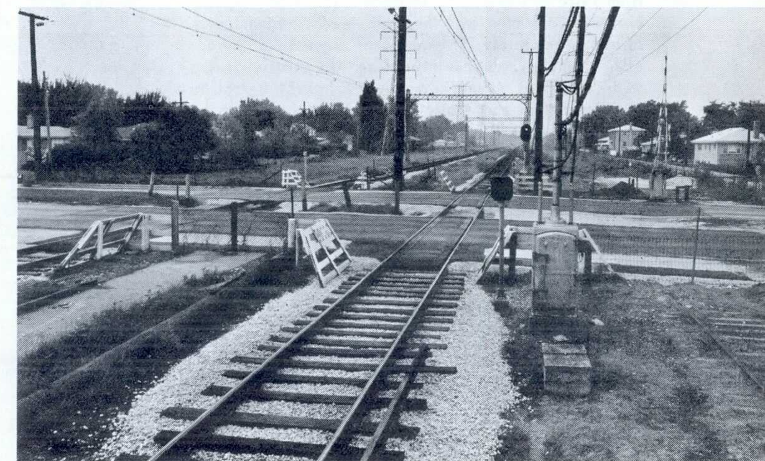
Tracks and pavement at Crawford crossing were completely rebuilt during the quarter to correct deteriorated conditions that had been reflected in excessive roughness for both trains and motor vehicles.
